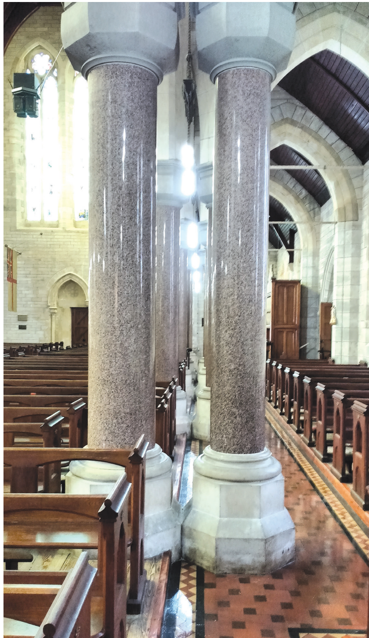
On the left: Trinity Cathedral has double columns down the nave for added stability during hurricanes.
